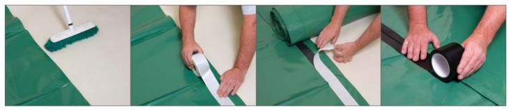
**1A** Unroll the first membrane, ensure the surface is dry and free from dust or grease. Inspect the membrane to ensure that there are no indentations or protrusions. If there are remove and apply sand blinding.
